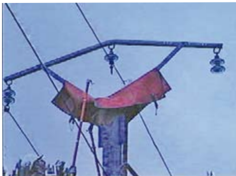
The holding in place of an insulating cover
